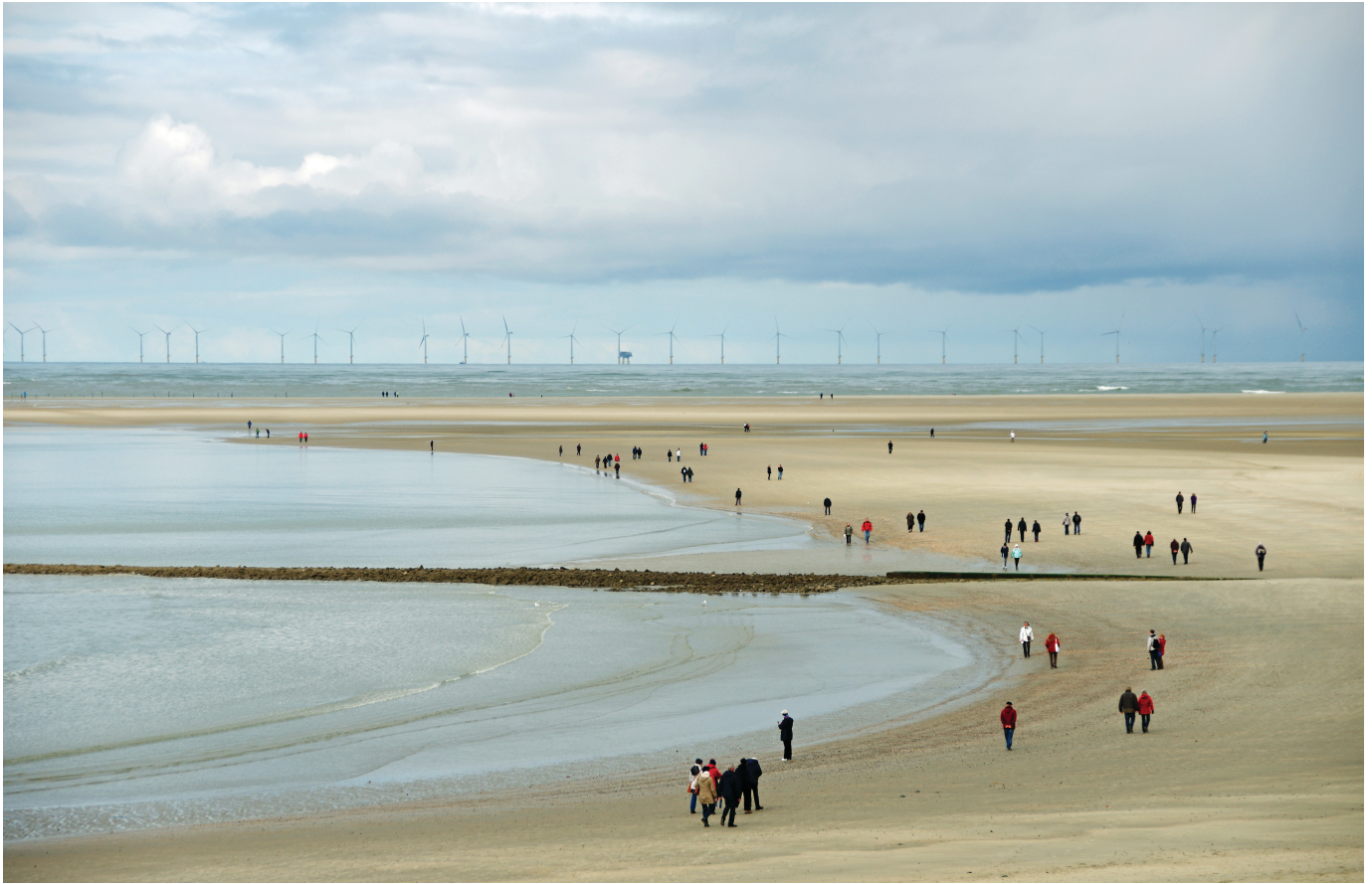
Off Shore Windpark. North Sea, Germany. PHOTO BY LUTZ KOCH
