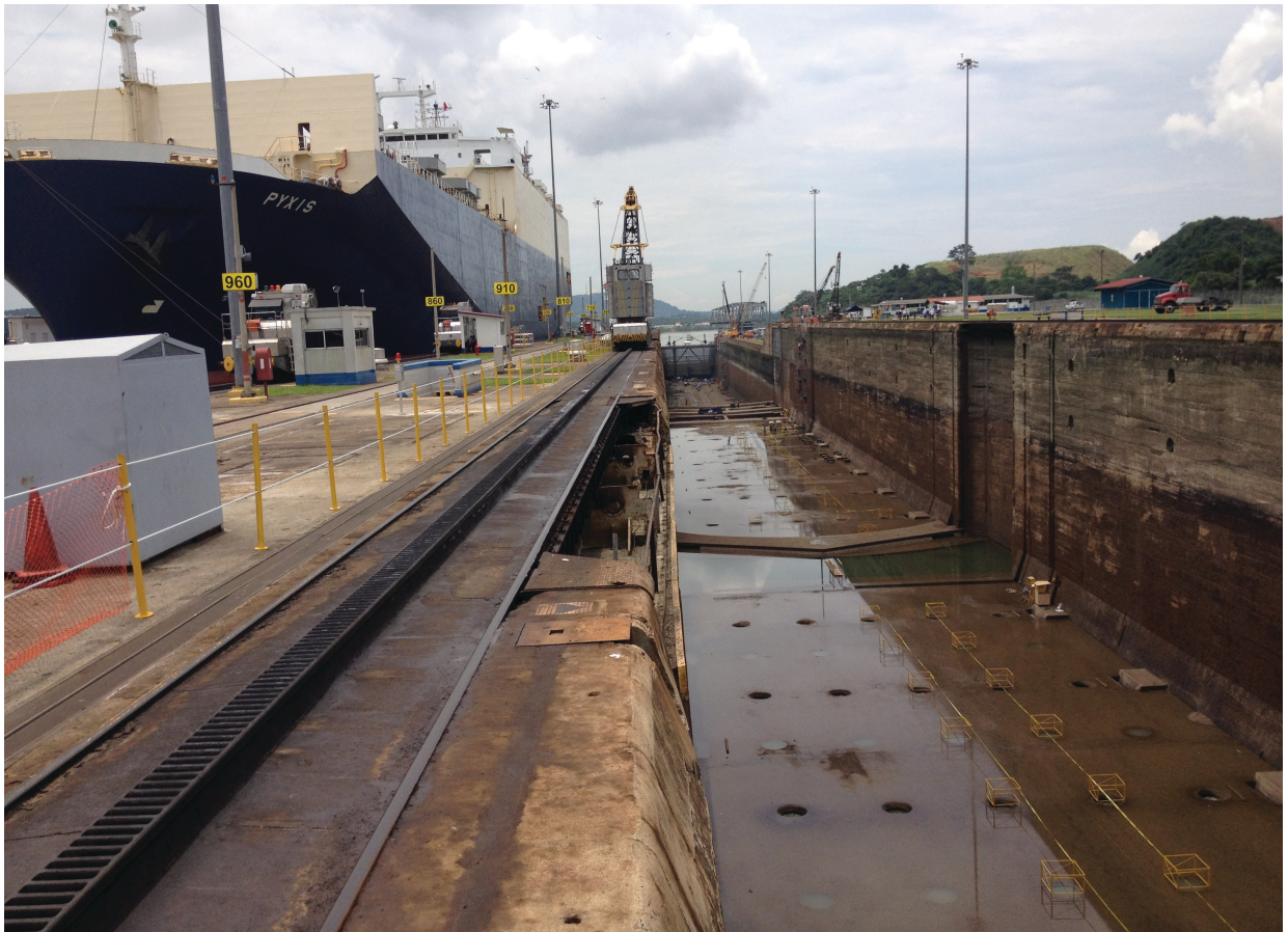
FIG. 4: The Panama Canal's locks require an enormous volume of fresh water to operate. Canal reservoirs also provide municipal water and hydropower for nearby cities (PHOTO BY THE AUTHOR).
