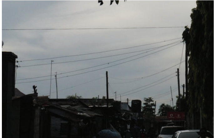
The service line assemblage. PHOTO BY FAISAL SHABAN
