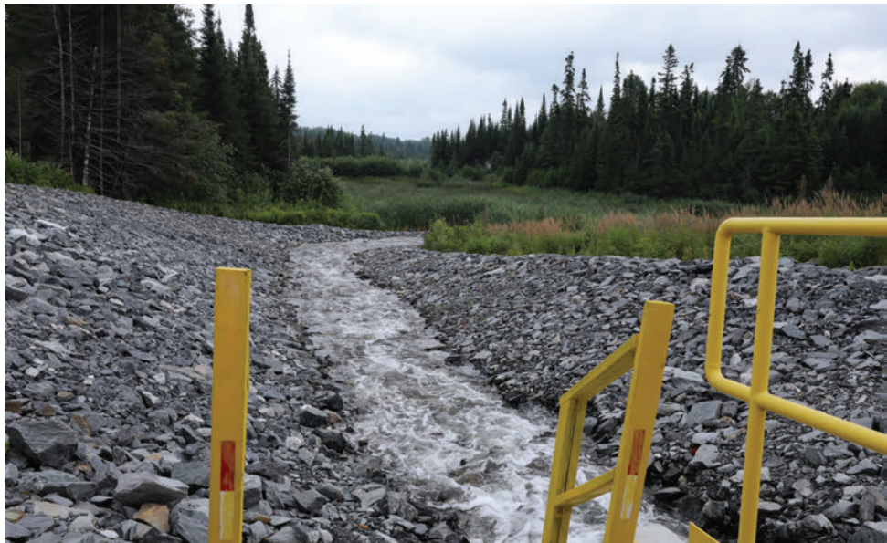
To avoid immediately killing wildlife, water from the mine must be treated to raise its pH from 2-3 to 5-6. Here treated water is released into the boreal forest. PHOTO: ORIT HALPERN
